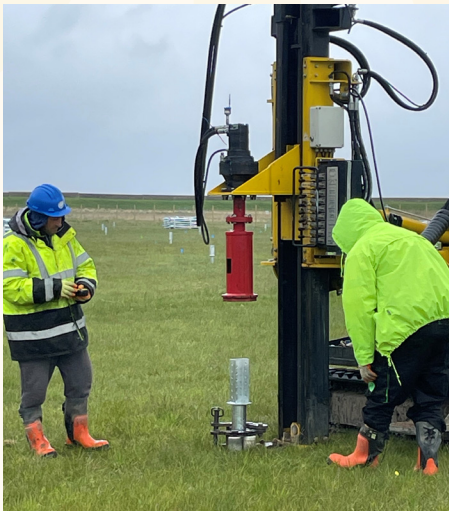
A two-man team installing screw piles
